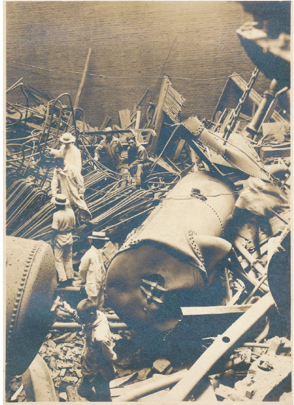
Fig. 6 Boiler explosion at Ajikawa Steam Power Station (1920) [12] (Courtesy of the family of Seiichi Ishigai).
